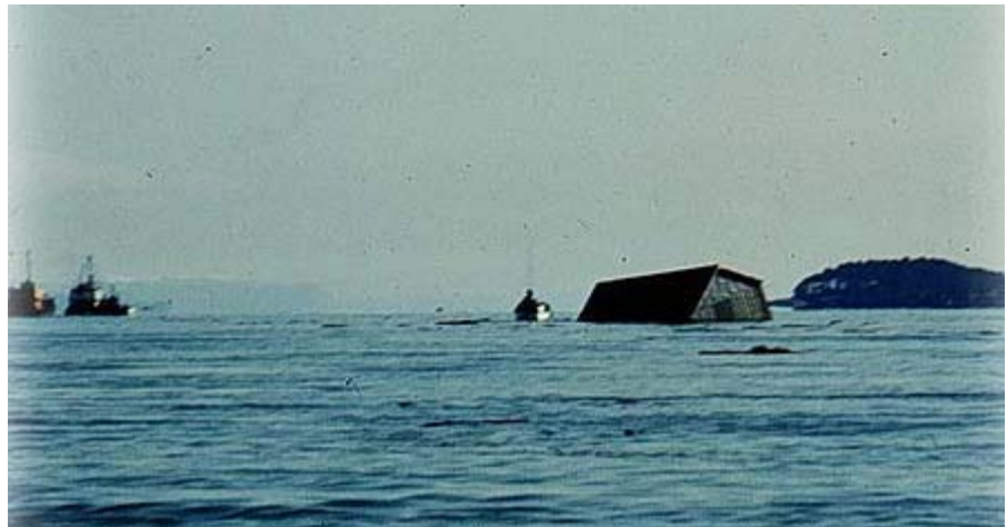
Fig. 7: The Afognak store was washed out into the ocean from the 1964 Earthquake and Tsunami
